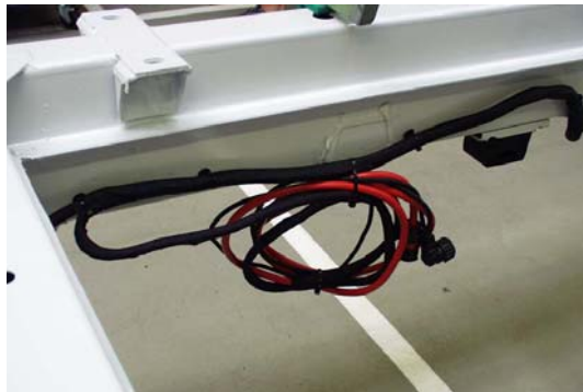
The plus cable and the connection to the cabin switch are fastened on the rear part of the vehicle chassis.
