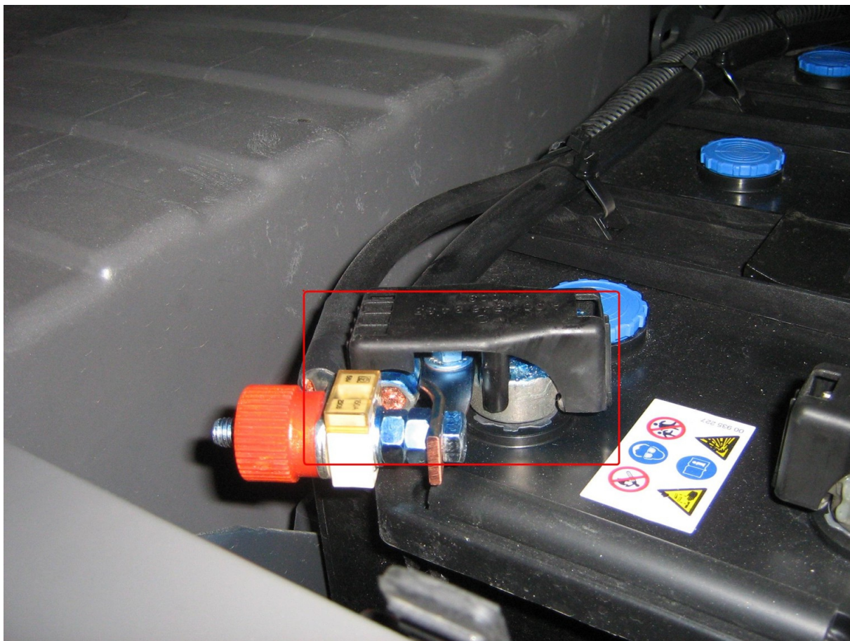
Package content so far: DB Atego battery clamp with tail-lift fuse
